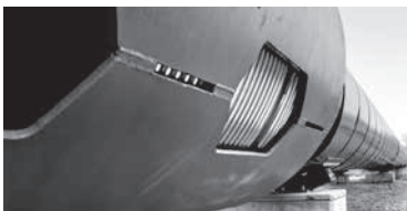
Fig. 12.13 Pressure balanced axial expansion joint, toroidal chamber principle, in district-heating pipe system DN 1000
